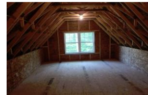
Future Bonus Room Framing
